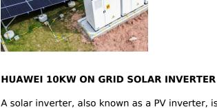
A solar inverter, also known as a PV inverter, is a type of electrical converter that converts the variable direct current (DC) output of a photovoltaic (PV) solar panel into a utility frequency ...
