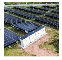
The plant will feature 29,600 solar panel modules with bifacial technology, which means that they will generate power on both sides of the panel. The plant's site covers the ...
