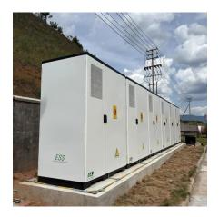
The battery energy storage system supported by the project is capable of storing 16 megawatthours of electricity and providing services to help with renewable energy integration, ...
